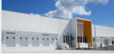
Industrial Ground-up Construction Homestead, FL
